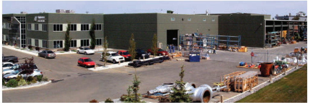
Universe Machine's 9,941 sq m (107,000 sq ft) operation boasts some of the latest in CNC machine tools including some of the largest machines in Western Canada.
